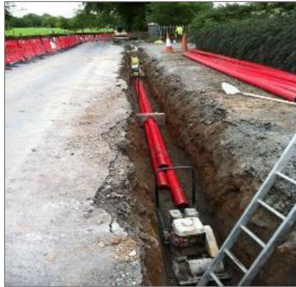
Figure 2 – Example of 110kV Underground Duct Installation
